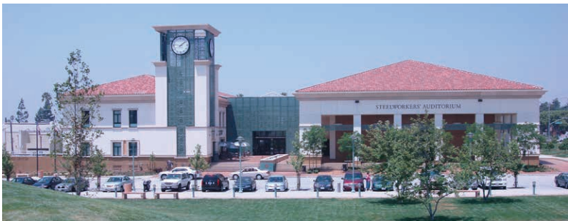
LEWIS LIBRARY AND TECHNOLOGY CENTER IN FONTANA - 2008
